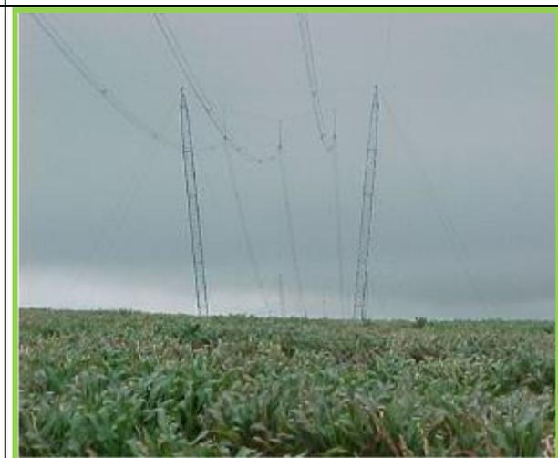
Figure 5: Cross rope suspension tower.
